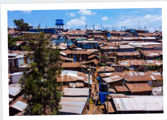
A SHOFKO-blue water tank stands high on the horizon overlooking Kibera informal settlements. Residents will gather at these tanks to access clean and affordable water for domestic use.
